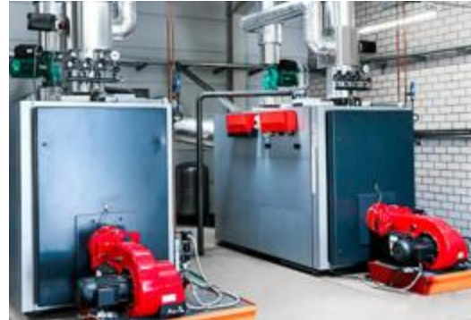
Diesel oil boilers replaced with more efficient gas condensing alternatives.
