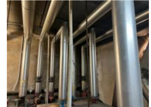
Installation of heat recovery systems for sanitary hot water at the air conditioning plant at the THB Guya Playa hotel.
